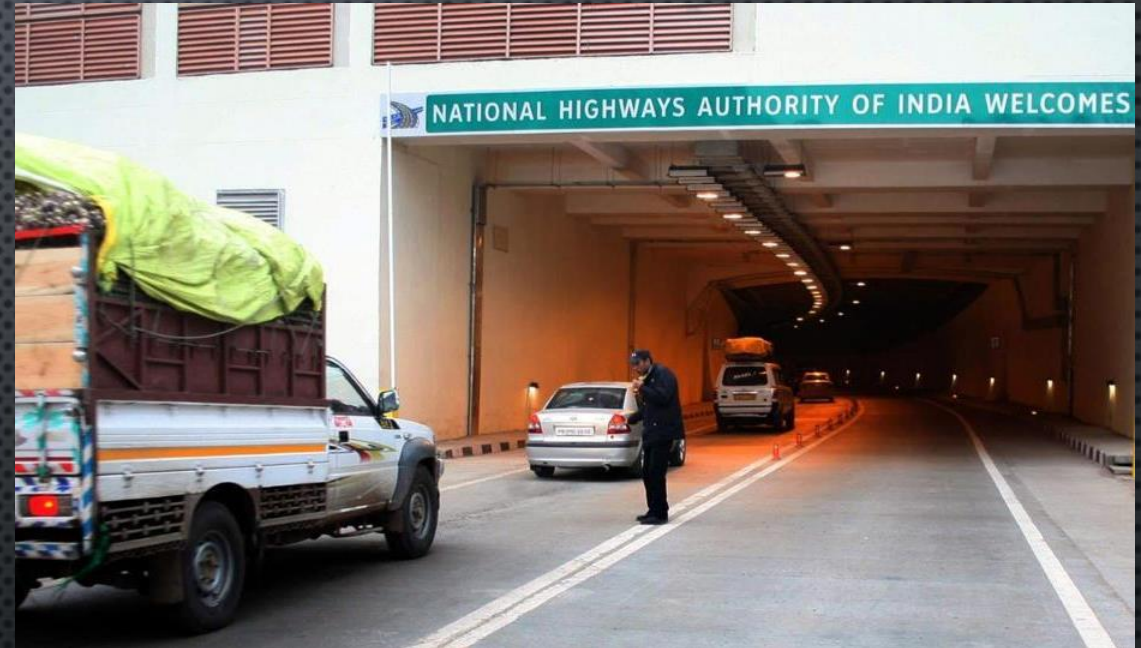
Figure 20: Chenani-Nashri tunnel connecting between Jammu and Srinagar [24]
